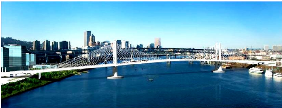
Overall Bridge View
