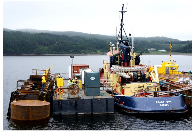
Assembled and launched limpet cofferdam ready to be positioned
