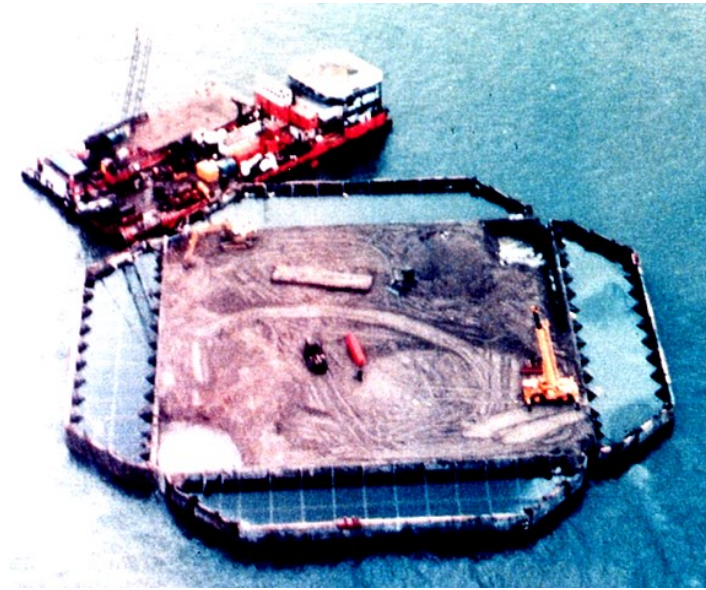
Landed caisson and beginning of dredge infill
