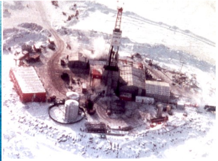
Completed island with exploration drilling in operation under full ice loading
