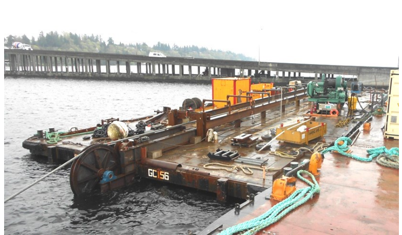
540-Ton capacity anchor test barge
