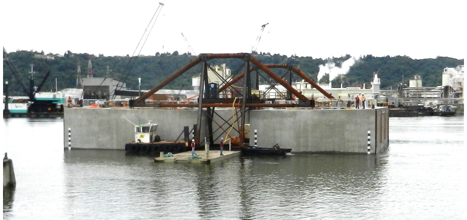
Pontoon Lift Barge in Service
