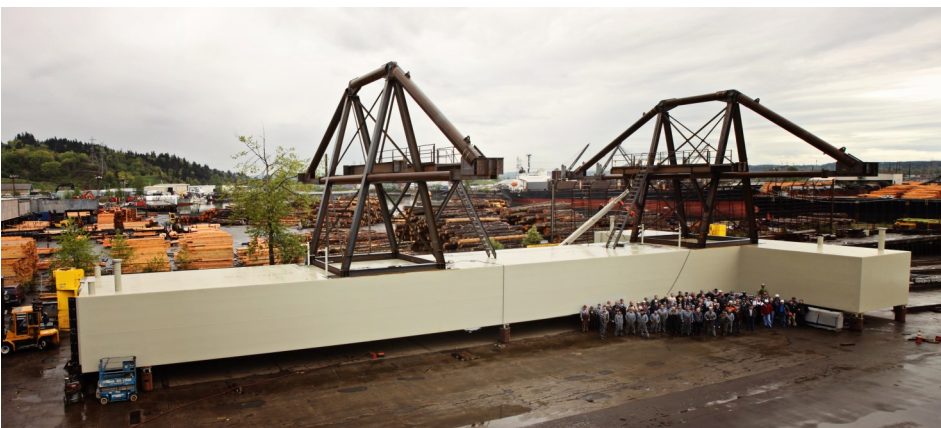
Pontoon Lift Barge Prior to Launch
