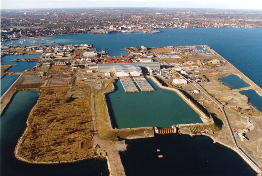
Arial view Oresund cast & launch facility in Copenhagen - Launching of 2 completed tunnel elements
