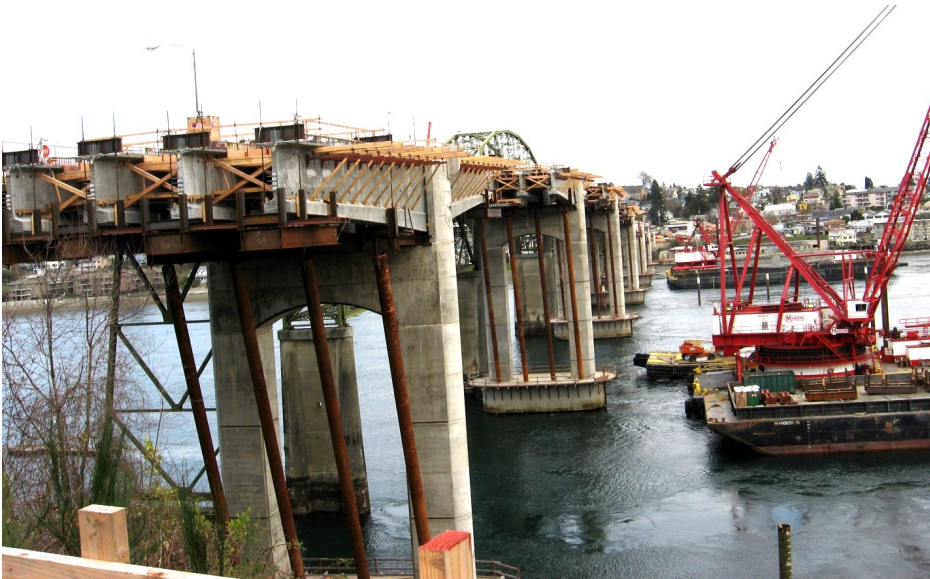
Lift-in precast pile cap cofferdams and spliced girder falsework
