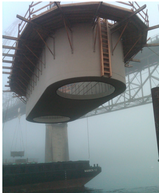
Lifting in of precast cofferdam
