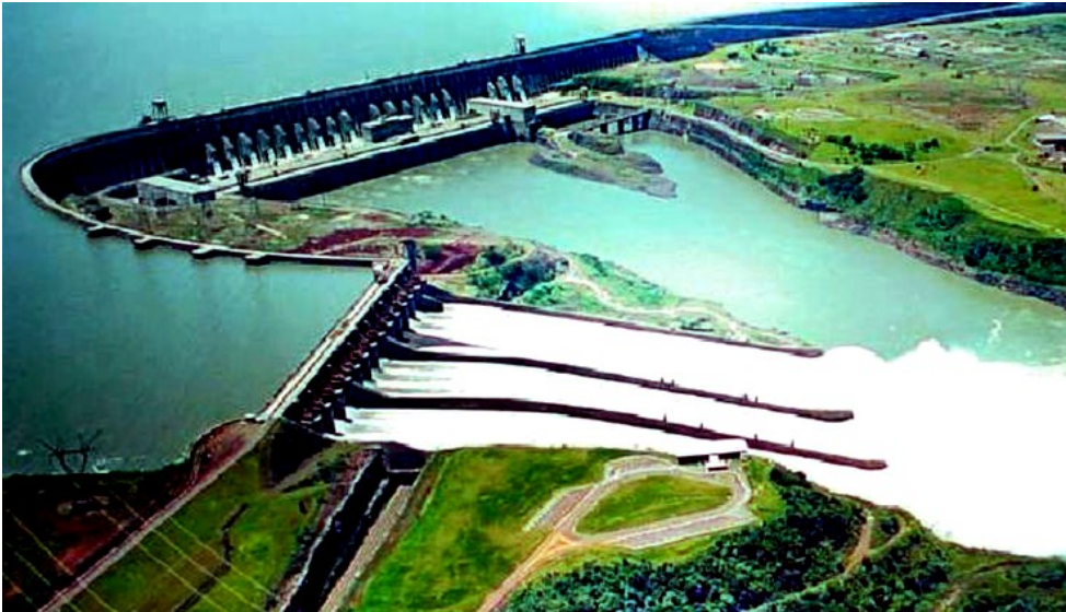
Completed Itapúa Dam in Operation
