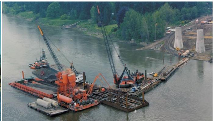
Placing 1200 CY tremie seal with floating batch plant
