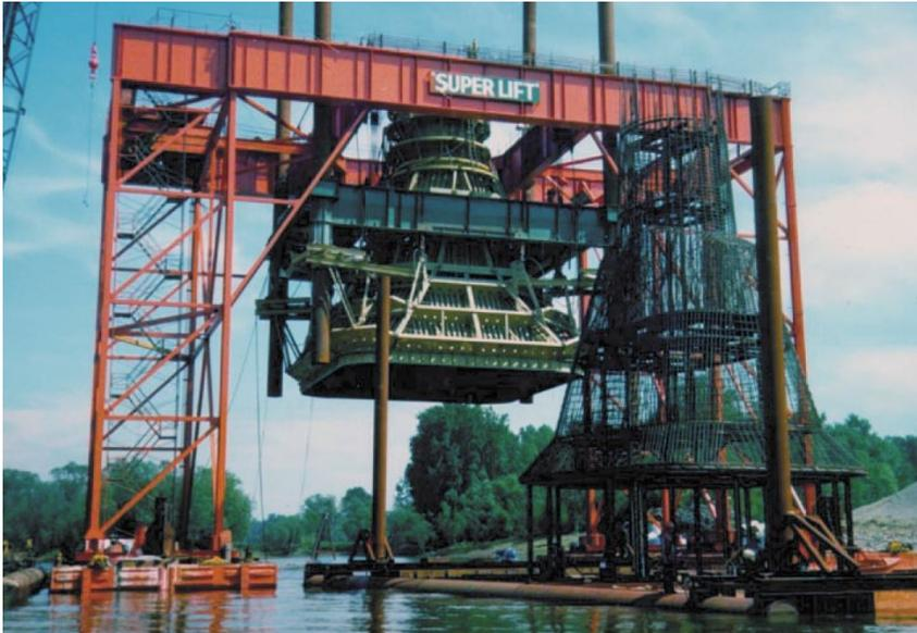
Bell shaped cofferdam mating to pre-fabricated reinforcing cage
