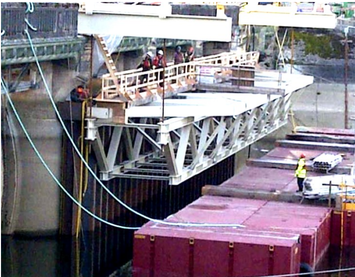
Installation of pre-assembled cofferdam
