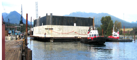
Pre-assembled cofferdam on 2 barges
