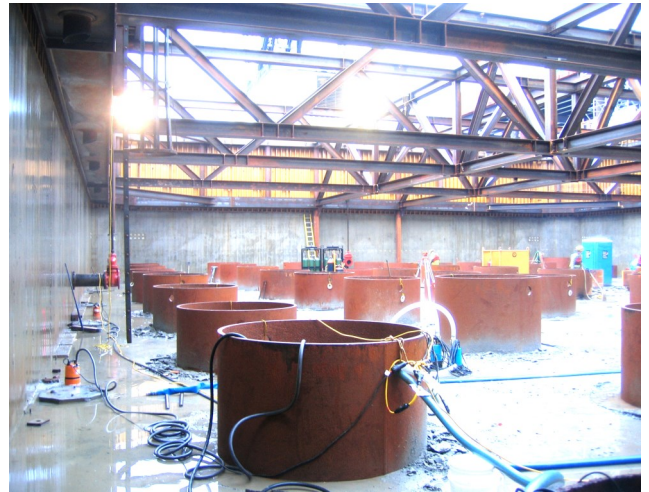
Interior view of the dewatered cofferdam
