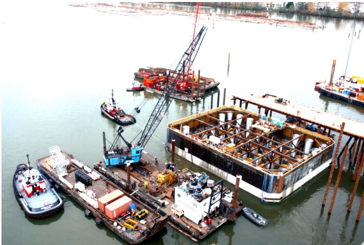
Floating cofferdam position in guide frame over piles
