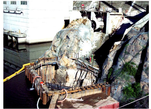
Aerial view of cofferdam prior to removal of rock dike
