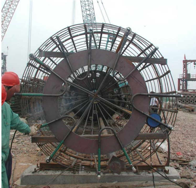
Figure 4 U-shaped grouting pipes at the shaft tip
