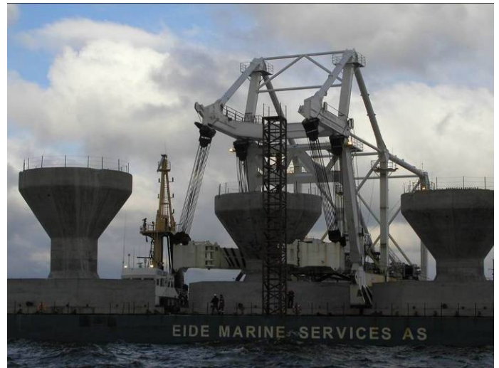
FIGURE 3 NYSTED OFFSHORE WINDFARM, INSTALLATION OF FOUNDATIONS (ABOVE AND BELOW)
