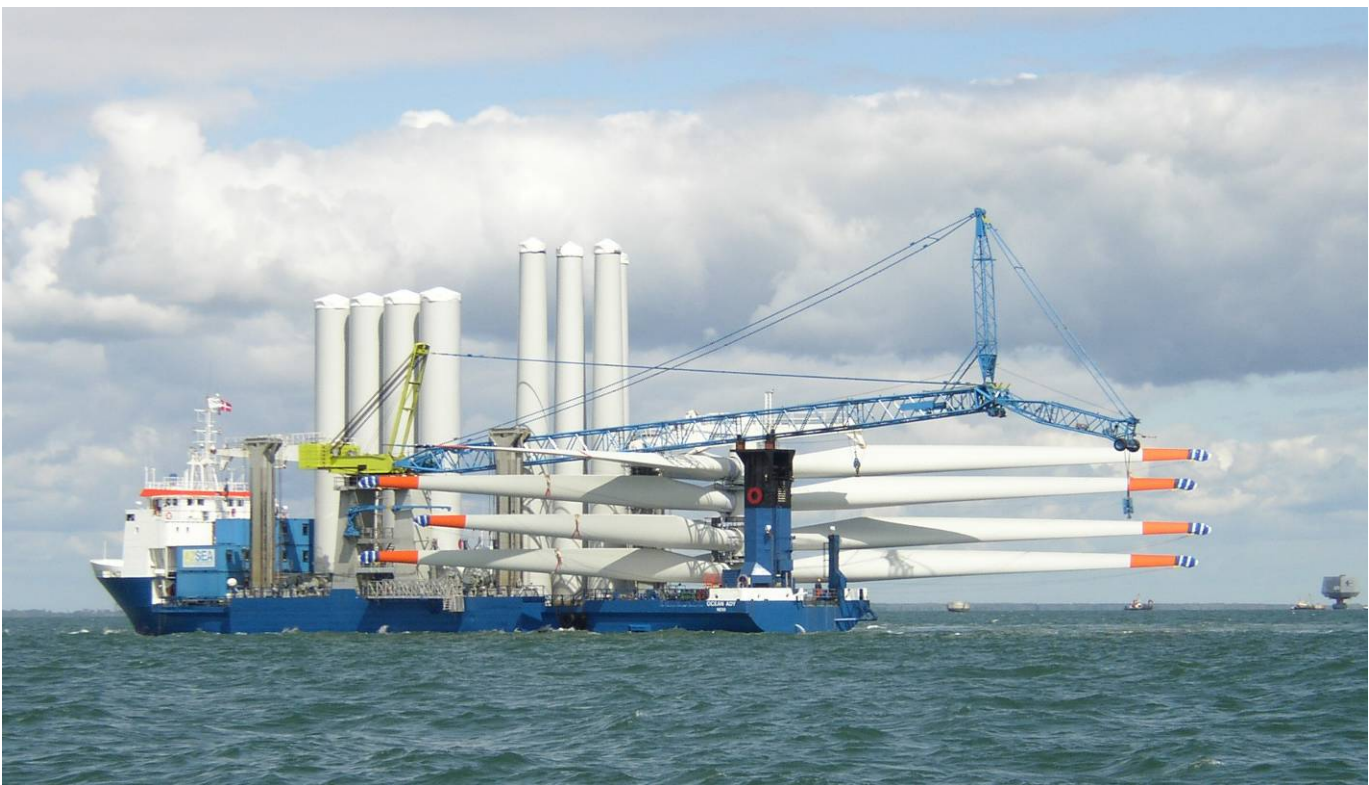
FIGURE 8 NYSTED WINDFARM, TURBINE INSTALLATION
