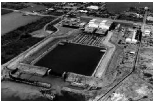
Figure 11 Two-level basin earth works and gates completed – temporary seaside dike is being dredged after successful test of gates
