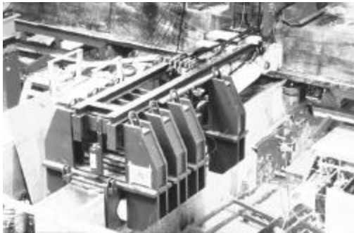
Figure 9 500 ton GTM pusher in action (22 tons in weight)
