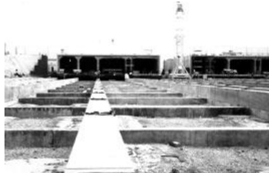
Figure 10 Reinforced concrete skid beams – view from shallow basin
