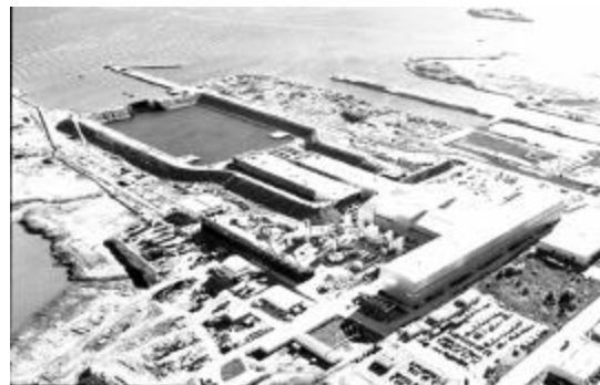
Figure 3 General view of site installations with its concrete batching plants close to the casting shed
