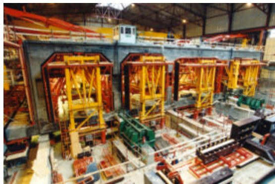
Figure 6 Steel form system for full section casting
