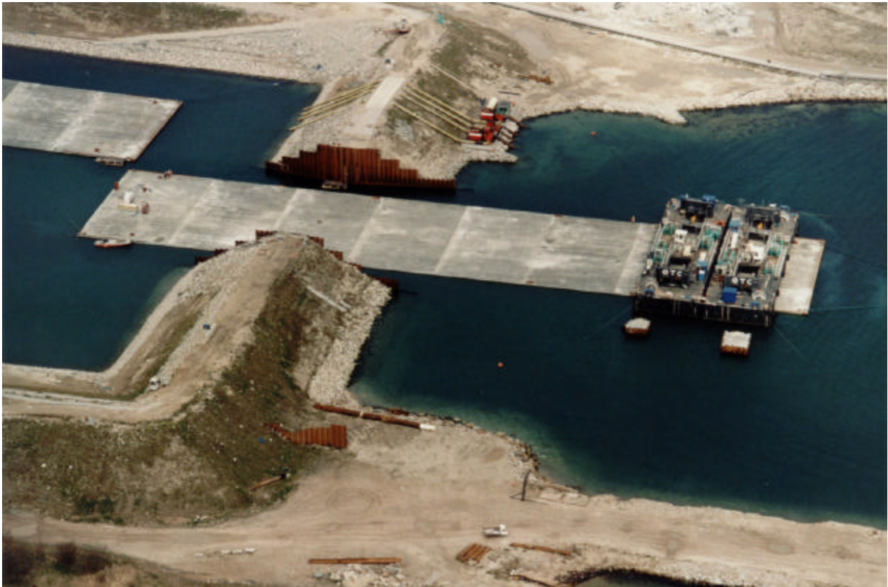
Figure 9 Completed tunnel element exiting the launch basin
