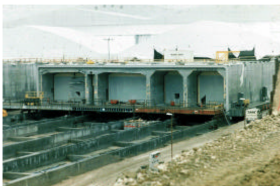
Figure 5 Element fabrication above sea level
