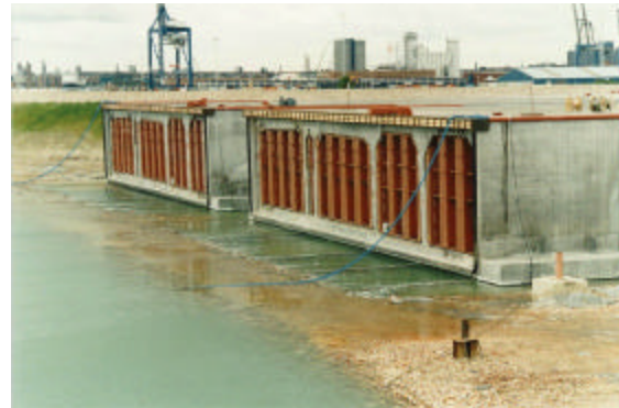
Figure 8 Crack free tunnel elements at time of launch
