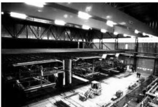
Figure 3 Completed reinforcing cage
