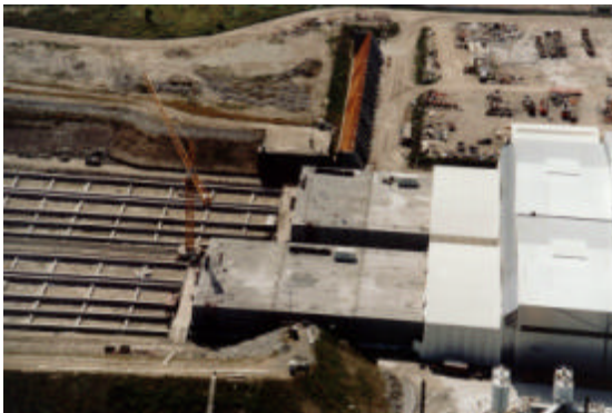
Figure 7 Hydraulically supported tunnel segments exiting the enclosed casting facility
