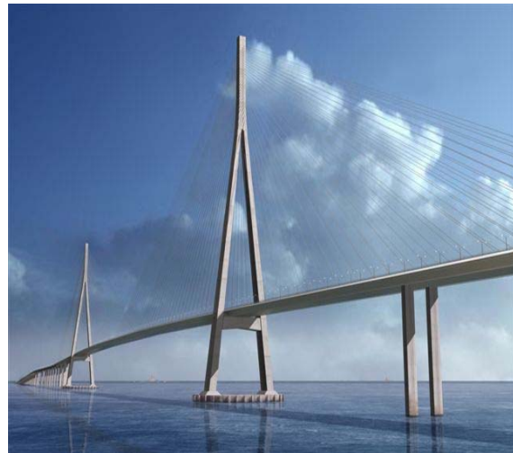
Figure 2 Sutong Bridge Main Span
