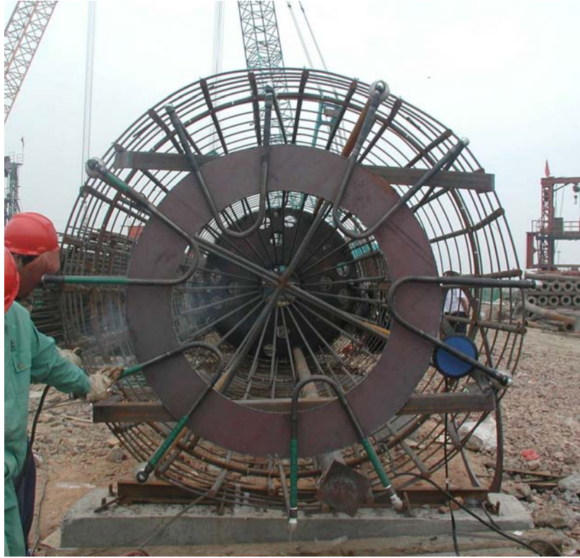
Figure 4 U-shaped grouting pipes at the shaft tip
