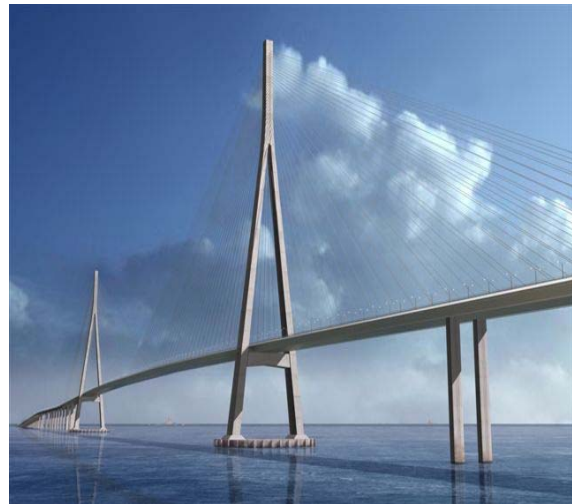
Figure 2 Sutong Bridge Main Span
